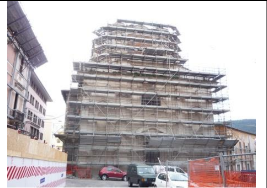
Photo4: Front View of Sant'Agostino dell'Aquila (under recovery works)
