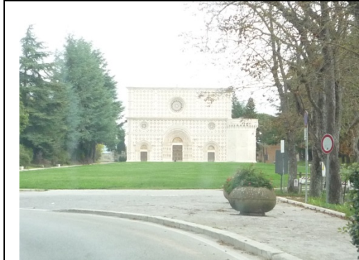
Photo3: Front View of Santa Maria di Collemaggio (under recovery works)
